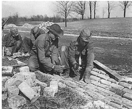
CCC Workers Constructing Road
