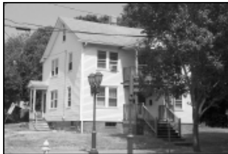
Dr. Hall House after inferior alter- ations 2005 (photo by Jane Bouley)
